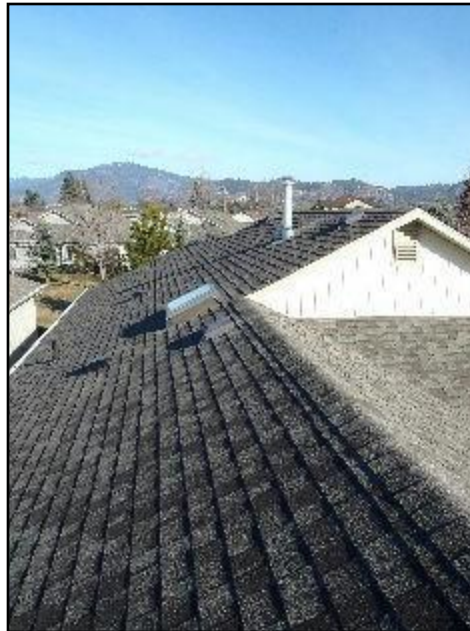
3. Asphalt shingles
