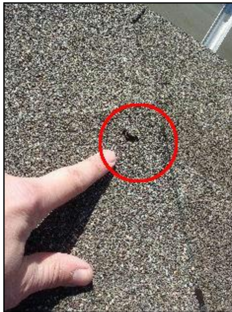
4. Exposed fasteners
