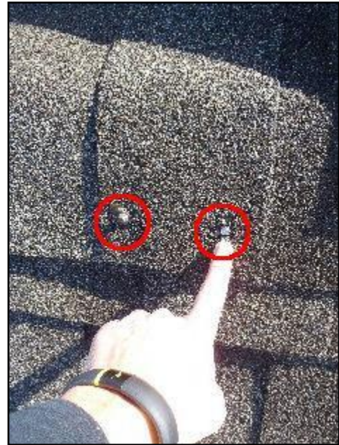
6. Exposed fasteners
