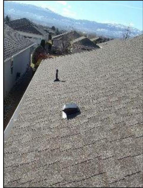
2. Asphalt shingles
