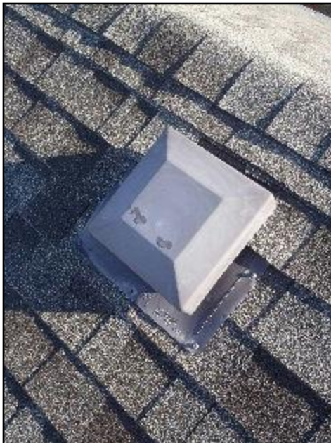
68. Roof and soffit vents
