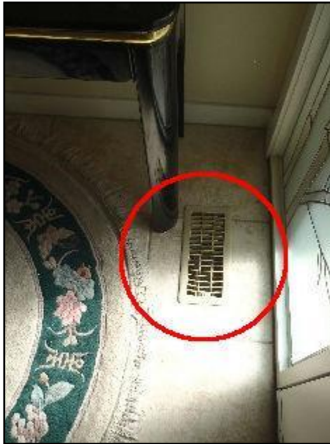
58. Ducts and registers
