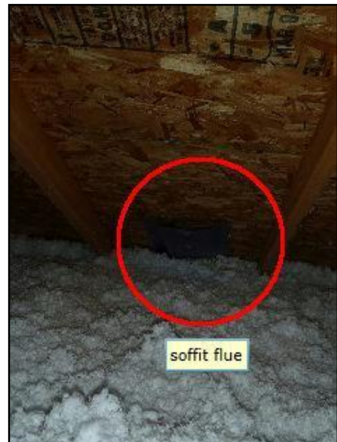
69. Roof and soffit vents
