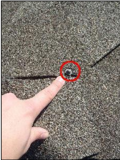
5. Exposed fasteners
