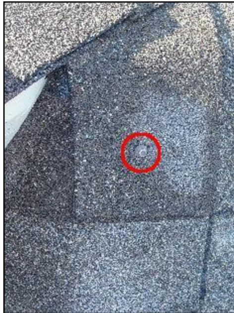
7. Exposed fasteners
